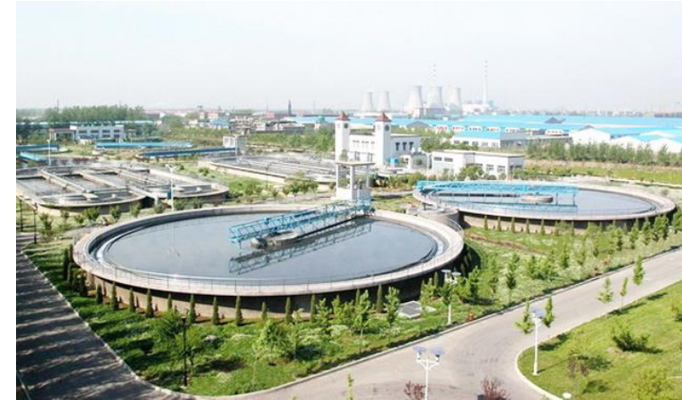
Fig 8. Sewage treatment plant in Huangjiahu, Wuhan province
