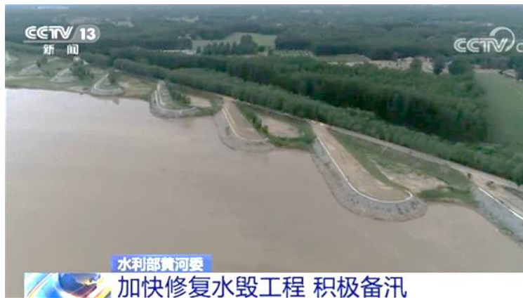
Fig 1. CCTV reported on the work about repairing damaged caused by floods
